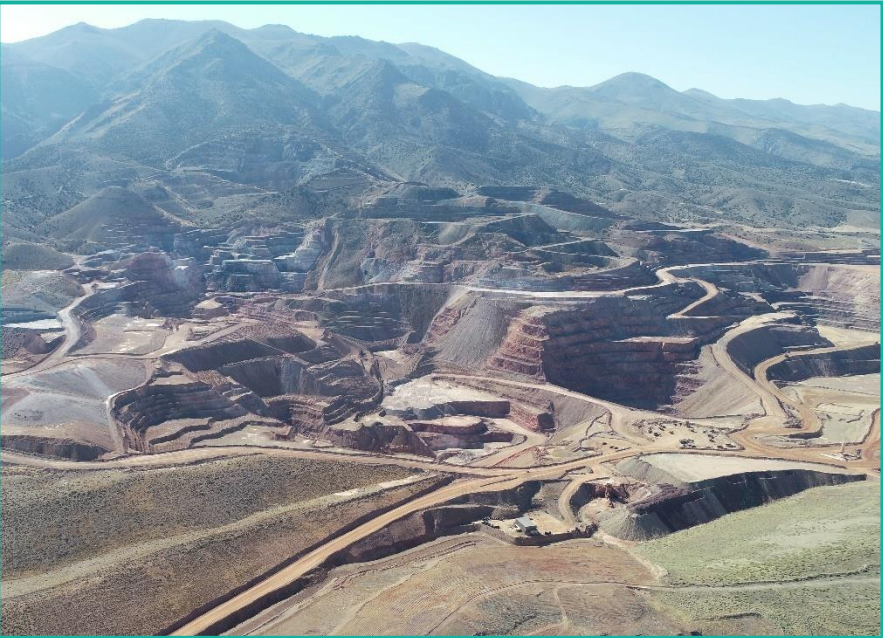
Site Arial View
