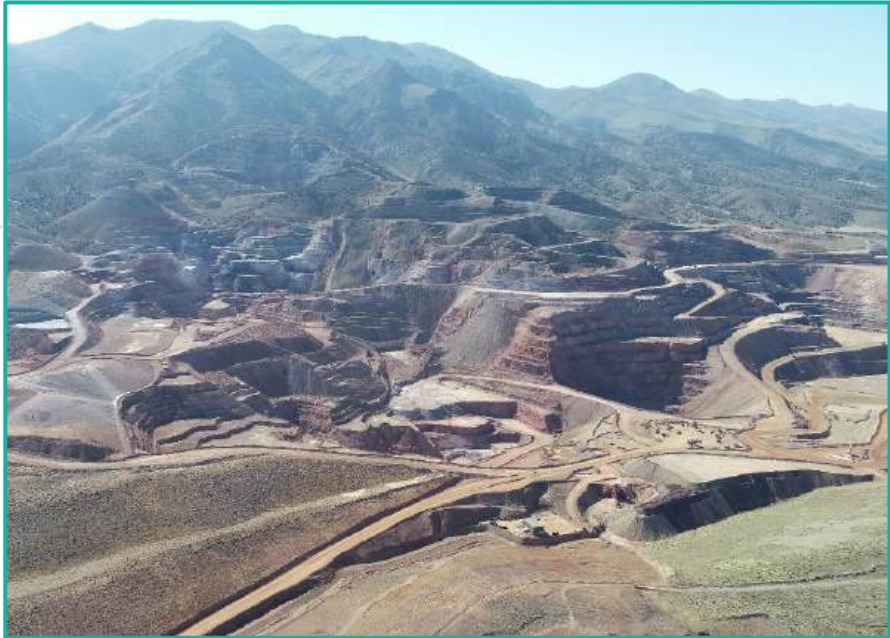
Site Arial View
