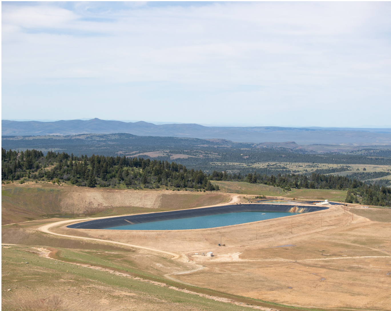
The DeLamar Project's water treatment facilities.
