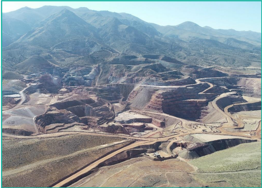
Site Aerial View
